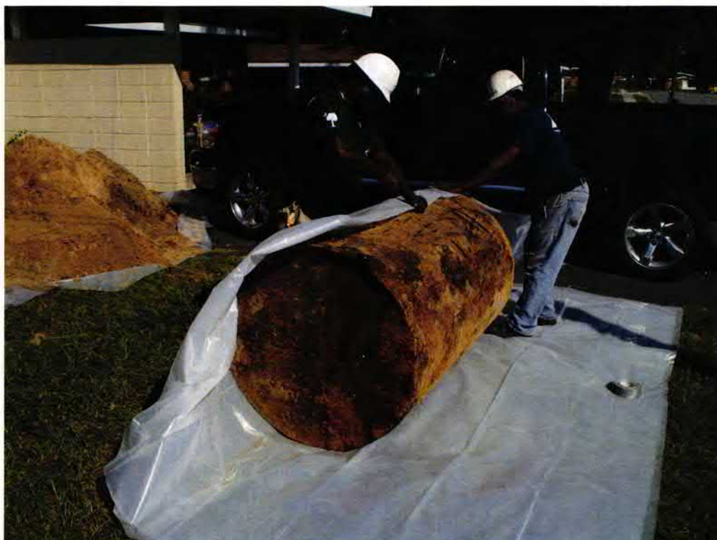
Picture 2: UST 1317 Albatross being wrapped for disposal.
